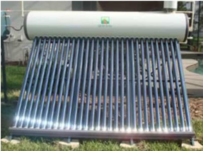
Solar water heating system (SWHS) is a device which supplies hot water at 60°C to 80°C using only solar thermal energy without any other fuel. It has three main components, namely,
